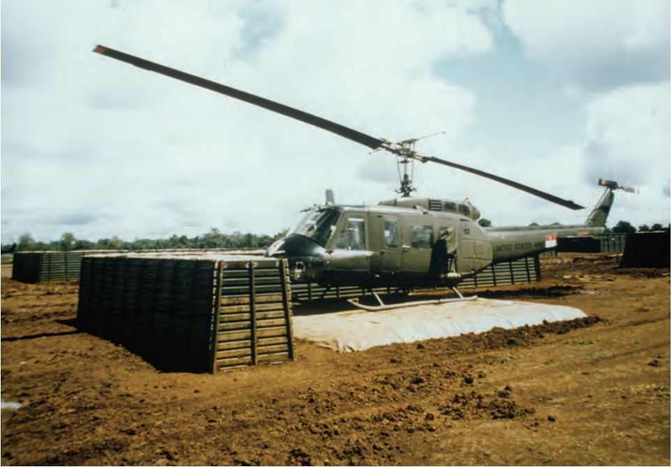
L-shaped helicopter revetment
